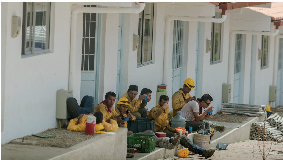
→ Workers eat lunch while working on the Nuevo Gramalote construction.
